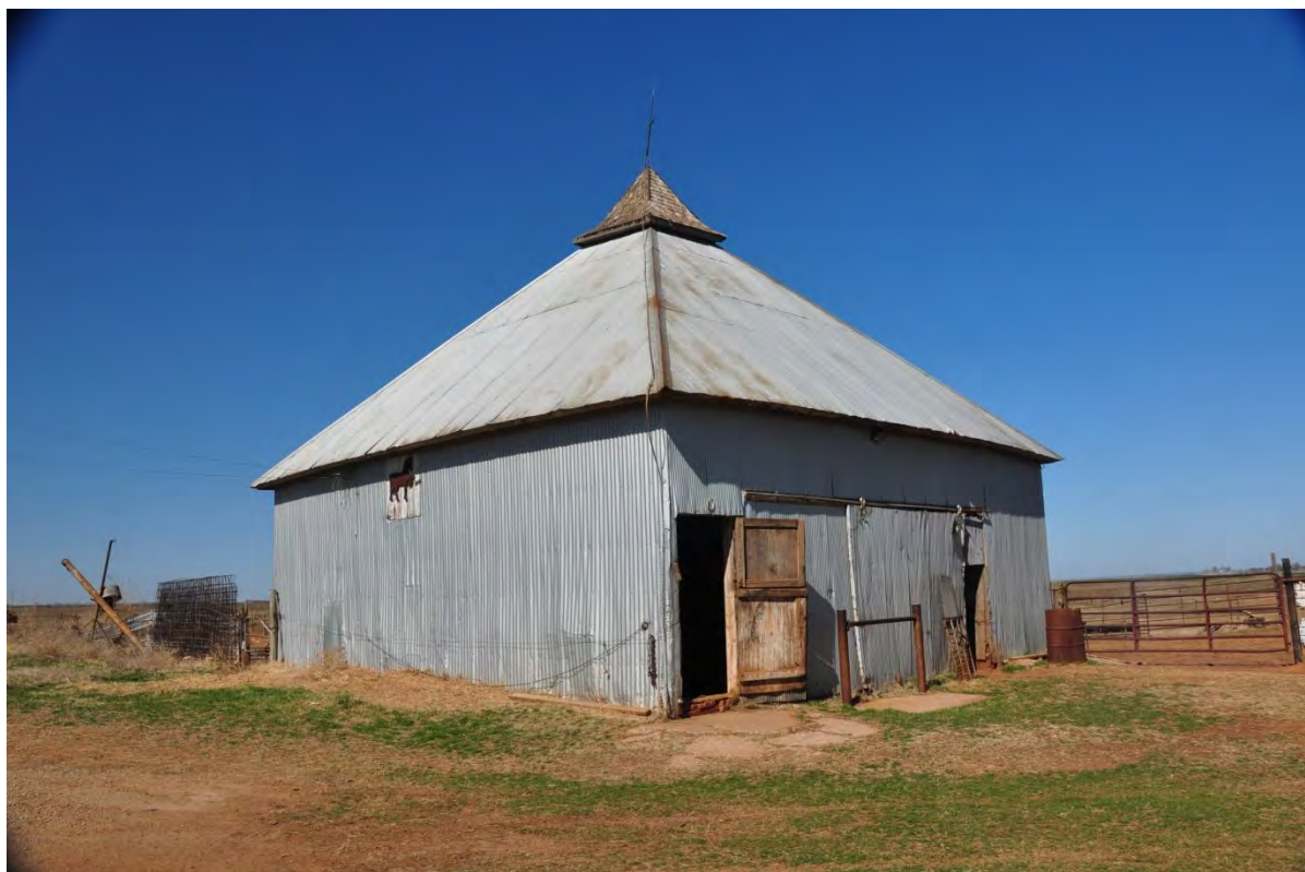
Parval square barn (1900), Nash vicinity, Grant County. This two-level square barn is one of three known to exist in Oklahoma. Note the hipped ventilator at roof apex.
