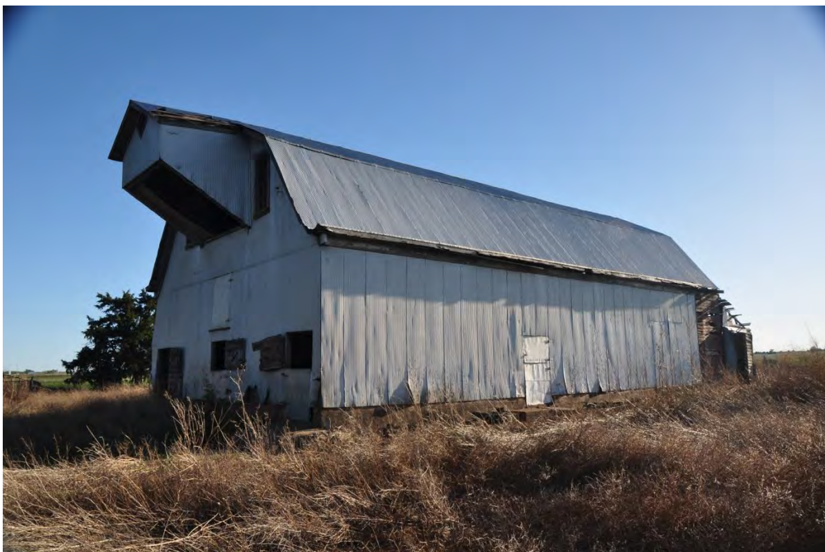
Large, boxed hay hood , Capron vicinity, Woods County. Larger barns designed to move larger amounts of hay sometimes have sophisticated hay hoods.
