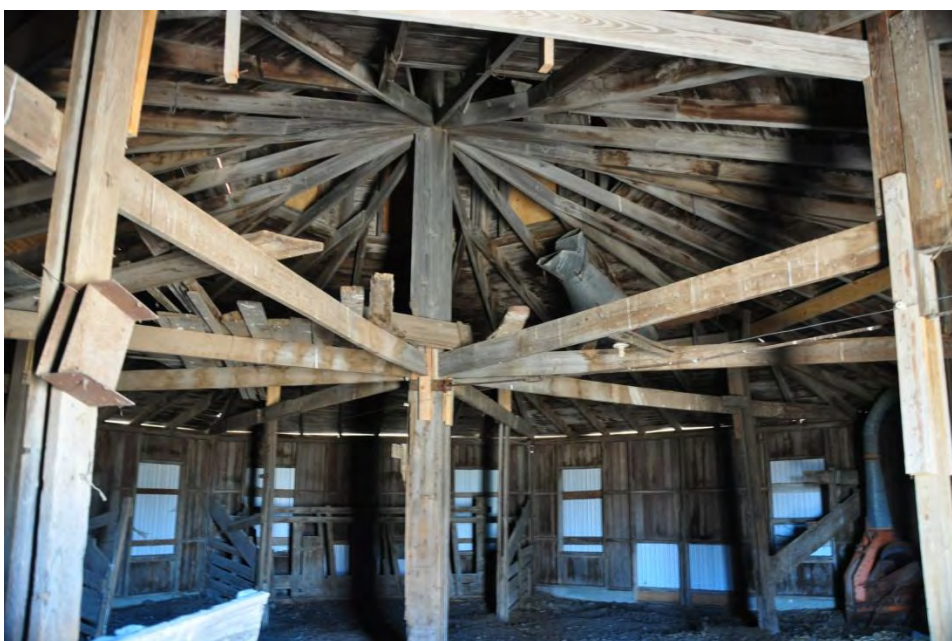
Octagonal barn under new sheet metal , Balko vicinity, Beaver County. The Slocum Barn, one of only three known historic nonorthogonal-plan barns in the state, is still used for local hog auctions. The recent addition of modern sheet metal, which preserves its functionality, greatly reduces its integrity and potential for National Register listing. Lower photo shows interior framing, milking stanchions and feed grinder.
