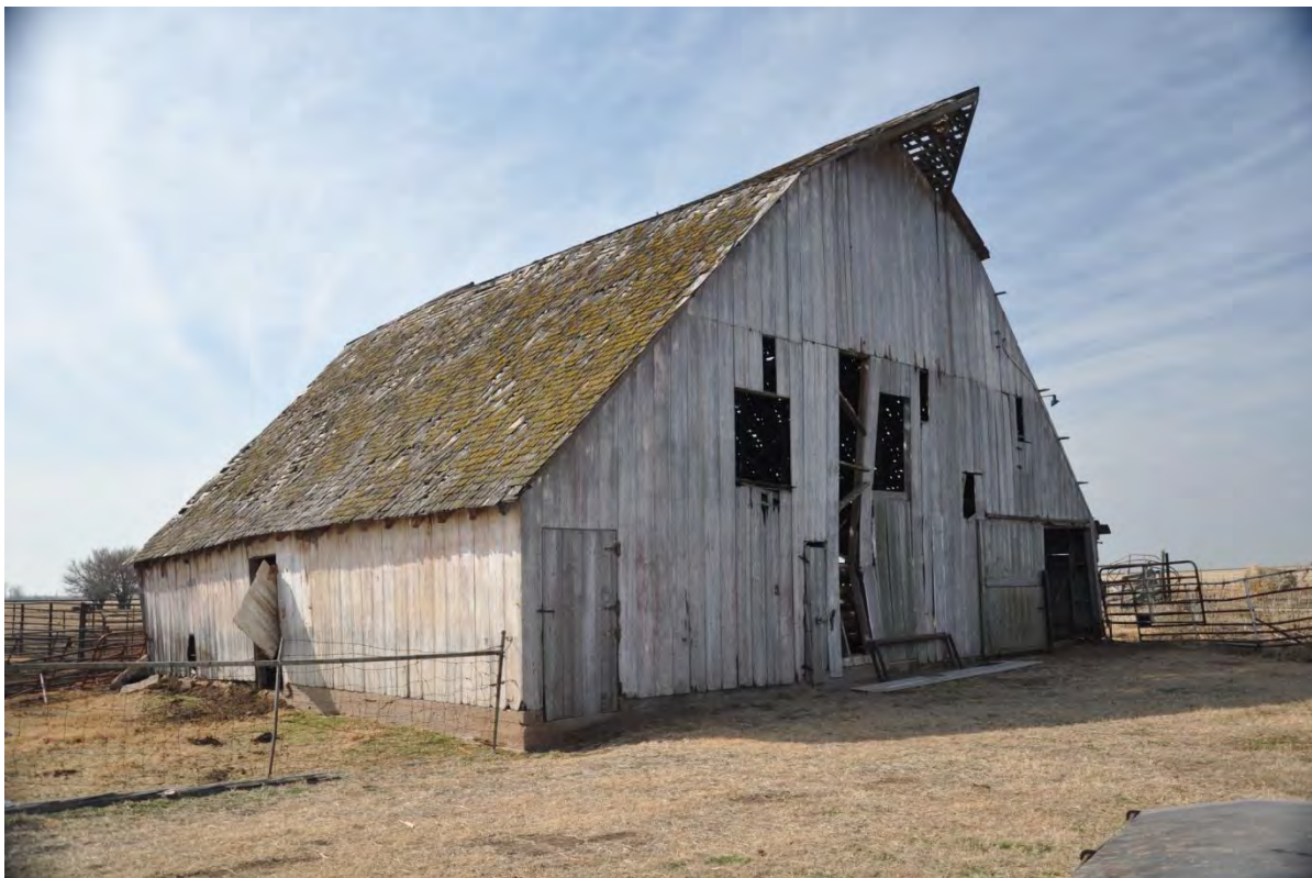
Godfrey Mack Barn , Salt Fork vicinity, Grant County. This relatively large, but otherwise typical barn was built in 1941 in the heart of the winter wheat belt of north central Oklahoma. Its floor plan conforms to that of the Midwest Three-Portal Barn described by Noble and Cleek, although it is classified here as a Midwest Livestock Feeder Barn.
