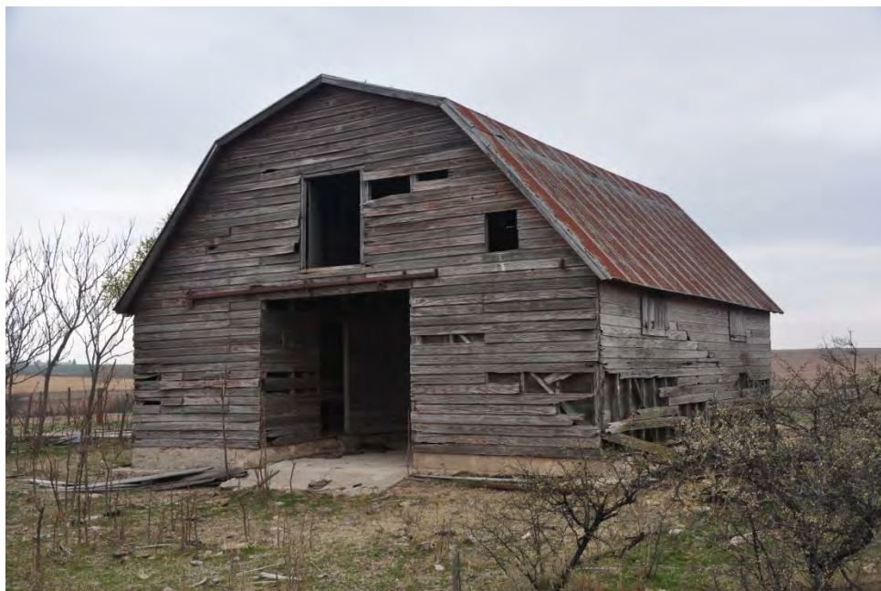
Transverse-crib barn, Shattuck vicinity, Ellis County. Note prominent center aisle.
