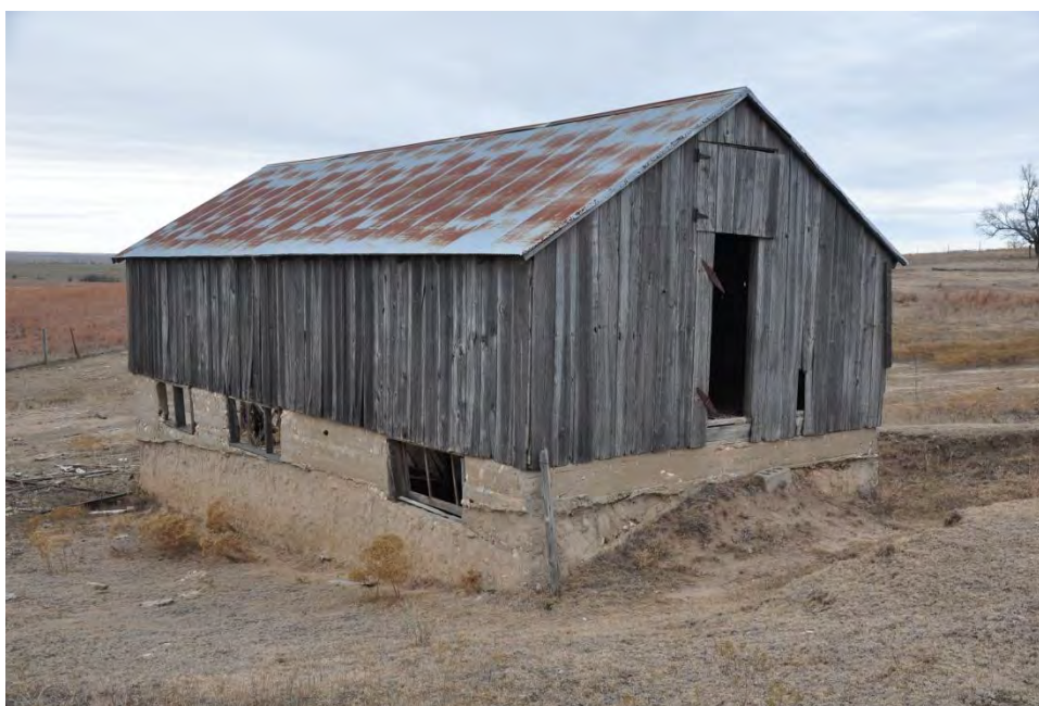
Gable-End Bank Barn , Catesby vicinity, Ellis County. Before the soil had so drastically eroded from this slope and the present owner removed the south doors (upper photo), hay was dropped through trap doors into the lower level, where cows were milked. This folk building has since been converted into a simple loafing shed for beef cattle. Remains of the earthen ramp can be seen on the opposite gable end (lower photo).
